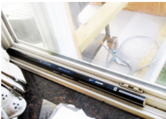
Figure 3. Salvageable Materials: The parts of this broken hockey stick were repurposed as a window-stoppers. Salvaging broken items often leads to an entirely new structure or system.
